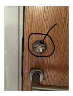
If you grab the door handle from the inside, the lock function is reset from the inside - this means that the door is not locked anymore. The door is now open from both the outside and the inside.
